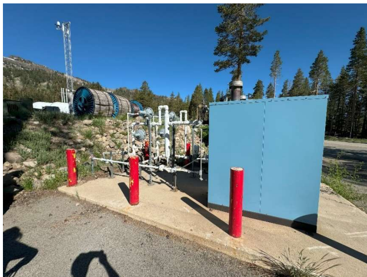
Figure 3.5: Existing Vaporizer (looking north)
