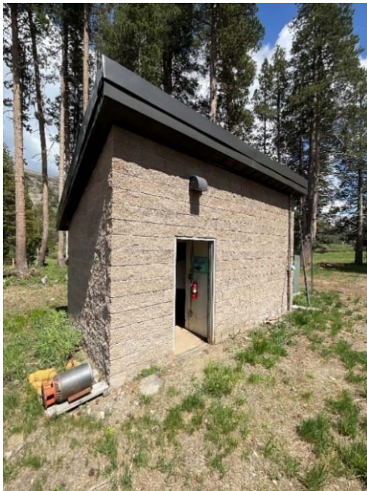
Figure 7-1: Well 3 Treatment and Booster Pump CMU Block Building
