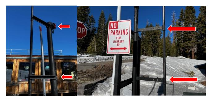
No matter how the hydrants are assembled, constant maintenance is required each year to keep the hydrants functional due to snow load (or snow creep) on the riser assembly.
