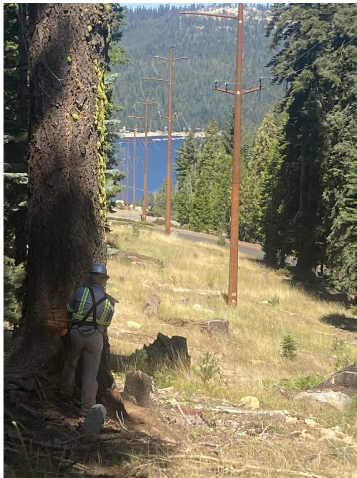
Figure 5 – 2026 Overhead Powerline Corridor
