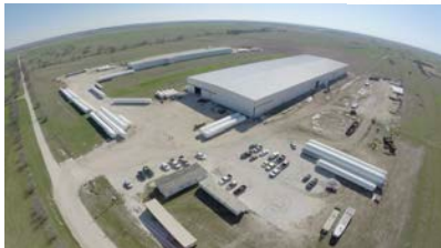
McGregor, TX 170,000 square foot fabrication facility TransTech Fabrication
