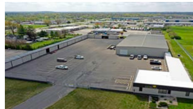
Indianapolis, IN 46,000 square foot fabrication facility Maddox Industrial Group
