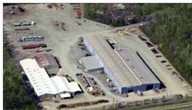
Charlotte, NC 65,000 square foot fabrication facility Bendel Tank & Heat Exchanger
