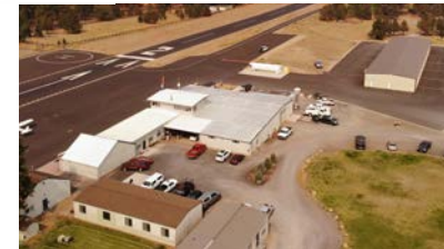
Sisters, OR 20,000 square foot fabrication facility ESI
