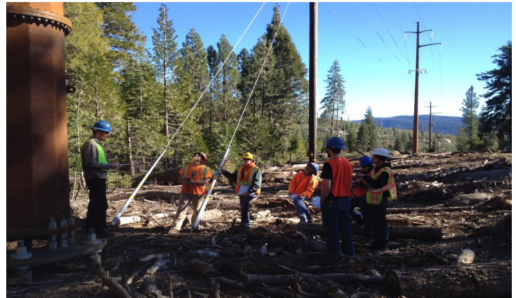
Training in progress on the Out Valley line
