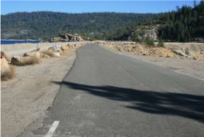
Photo 5. Segment 3. View south across FS Road 8N03 on Bear River Dam.
