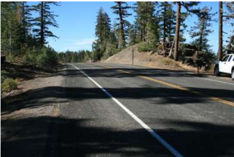
Photo 18. Segment 6. View west of Hwy 88 from near Maiden's Grave. Alignment would be on the north side (right) of Hwy 88 ROW.
