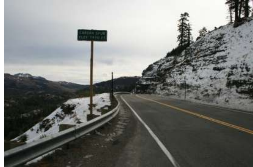
Photo 35. Segment 20. View east from Hwy 88 of Carson Spur.
