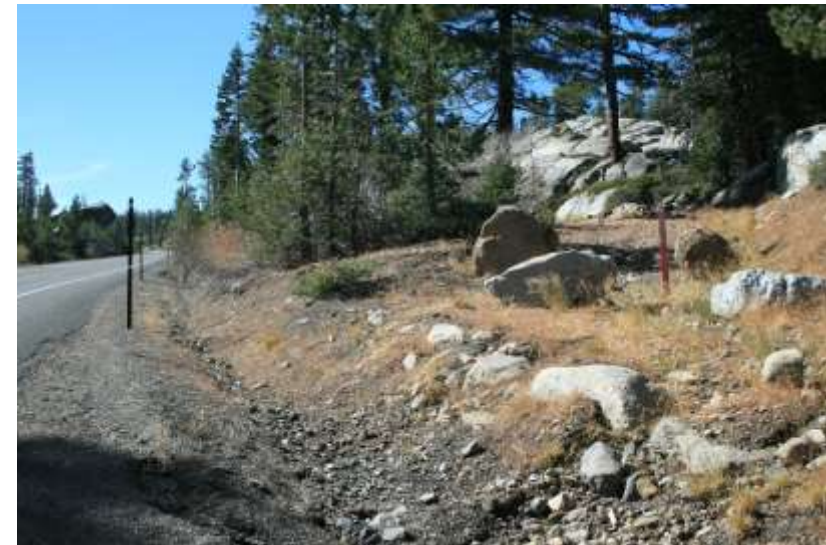
Photo 24. Segment 10. View of Volcano Optic Cable ROW near Hwy 88. Orange "call before digging" warning post can be seen.
