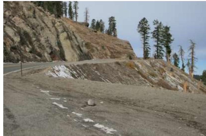
Photo 36. Segment 20. View west from Hwy 88 at Carson Spur.
