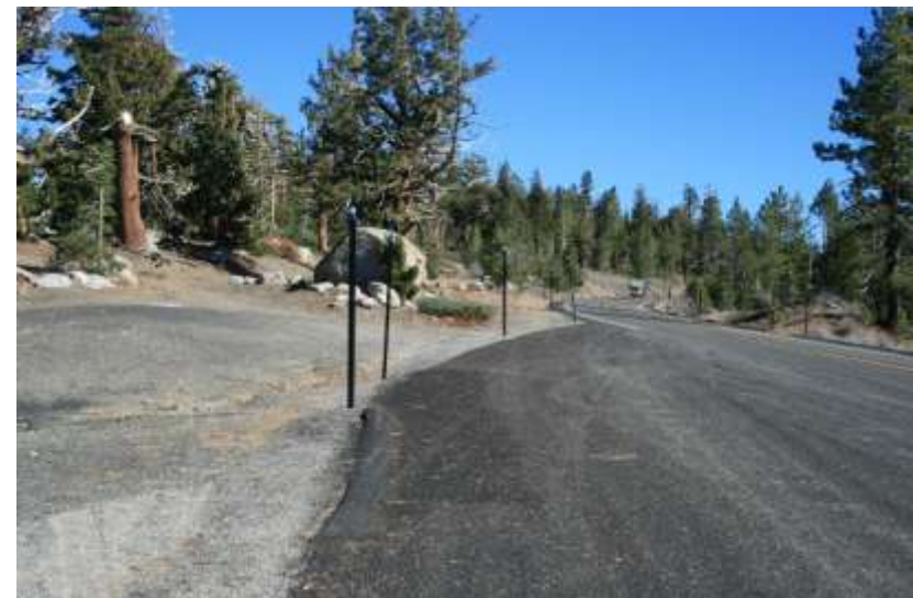
Photo 20. Segment 7. View west of Hwy 88 at Devil's Garden Vista Point. Alignment would be in Hwy 88 ROW on north (left) side of road.
