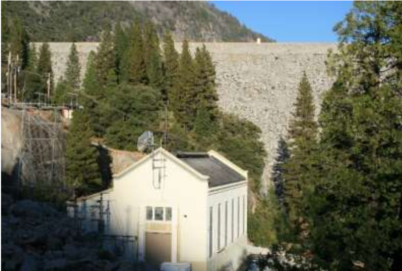
Photo 1. Segment 1. View of Salt Springs Powerhouse Area. Existing PG&E 21 kV line is coming down hillside on the left.
